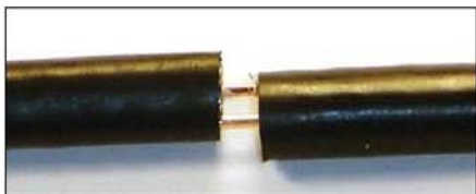
Figure 6 — The final joint with gap of about \frac{1}{8} inch. Take care to clear away any wire strands or bits of foil from the center conductors.
